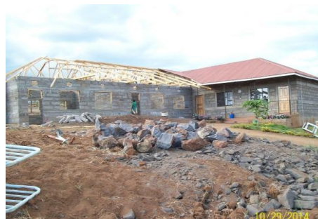
Classroom under construction at St. John Vianney Orphanage
